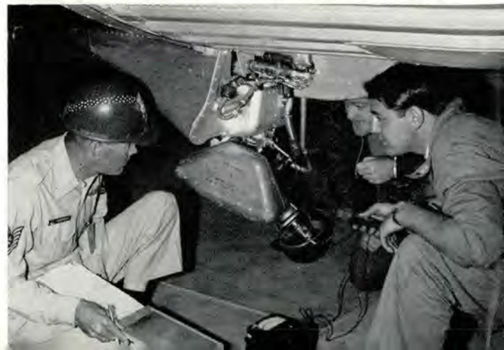
Sgt Jeffers and CONVAIR technicians conduct stray voltage checks on the bird prior to connecting the igniters. Here, Sgt Jeffers verifies "no voltage" on the vernier engine igniters of the Atlas.
